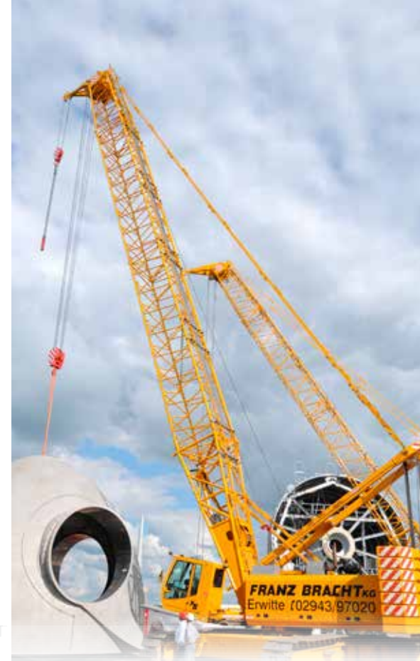
Top: Lattice boom crawler crane deployed in the installation of a wind power station.
